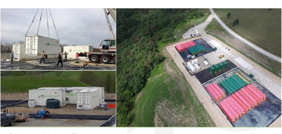
Onshore, produced water Treatment. 1500ppm inlet to < 1ppm outlet. Removal efficiency of 99.9%
