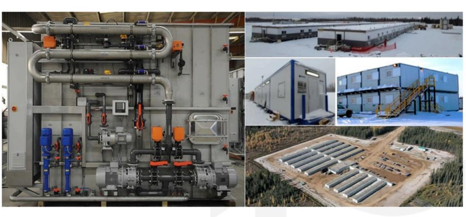
Remote man-camps in Alberta, Canada. Grey waters are recycled and meet local discharge regulations. The WaterPaqs are fully winterized with full redundancy in the control system
