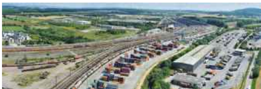
CFL multimodal, Bettembourg
