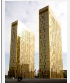
Civil Construction & Infrastructure Projects
